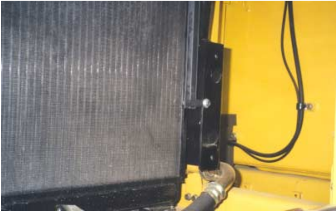
Right side lower condenser bracket with spacer behind intercooler bracket.
