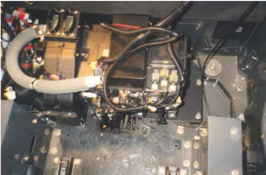
Evaporator assembly mounted in place.
